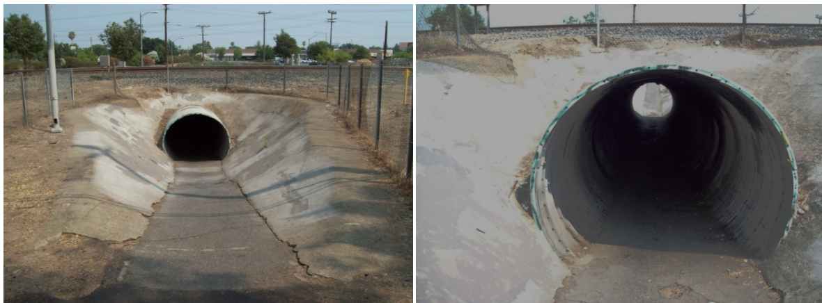
Figure 3: Entrance to the existing CMP ped/bike underpass
