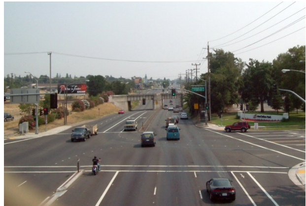
Figure 2: Existing Watt Ave UP looking to South
