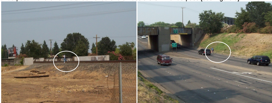
Figure 4: Cyclists avoiding the CMP underpass are a significant safety concern
