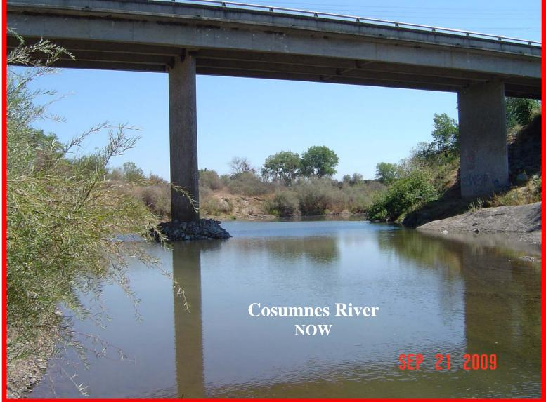
Structure Description: T-girders (4), continuous on RC piers, and on RC diaphragm abutments
