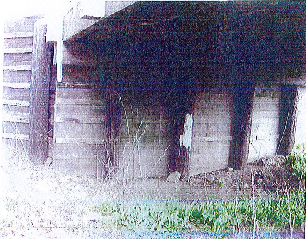
Photo No. 3 Abutment 17.
